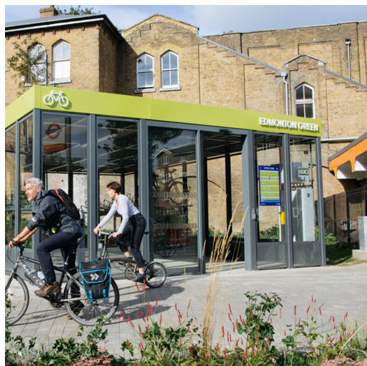
Integrated bike parking as part of the mobility hub facilities
